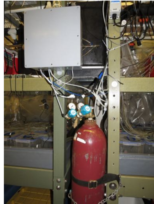
Carbon Dioxide Tank
